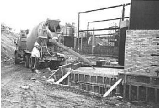
Fig.3 Application of EABASSOC Foamed Concrete
