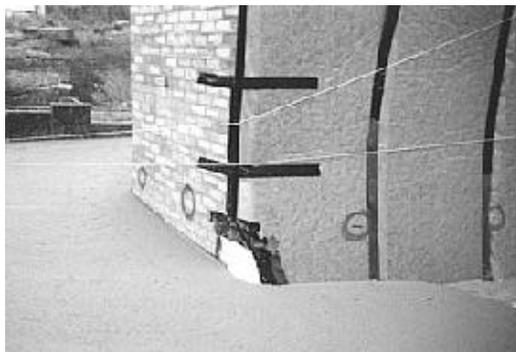
Fig.4 EABASSOC Foamed Concrete after application
