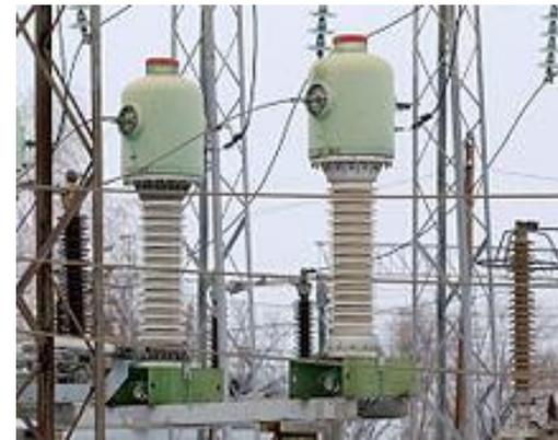
SF<sub>6</sub> 110 kV current transformer TGFM series, Russia
