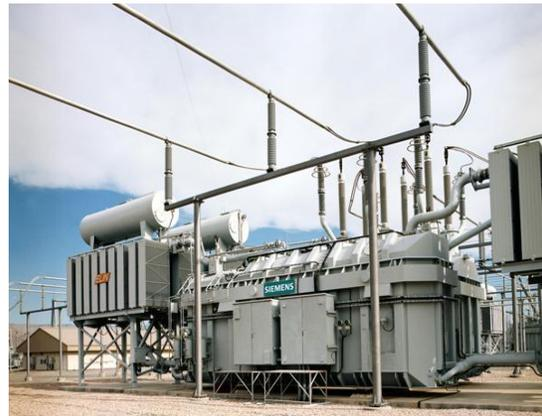
Phase shifting transformer for power flow control
