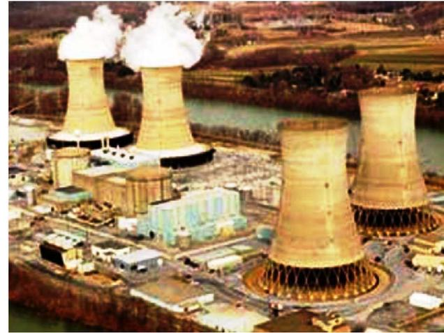
In nuclear power station, Uranium ( $U_{235}$ ) is subjected to nuclear fission in *nuclear reactors* (breaking nuclei of heavy atoms into two parts with release of huge amount of energy) . Consequently, released heat energy raises steam's temperature and pressure.
